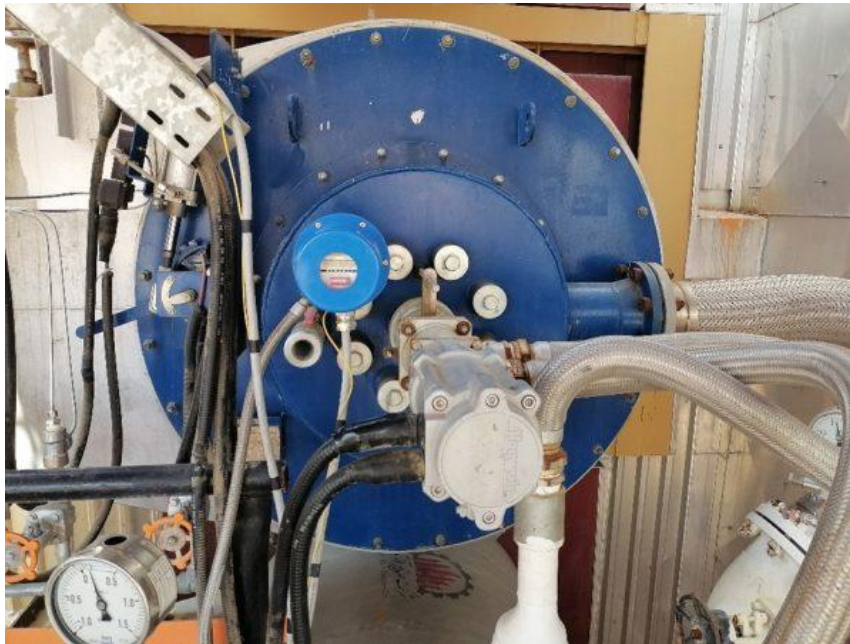
Installing NoorParto's flame detector on the boiler of the Bidblond refinery
